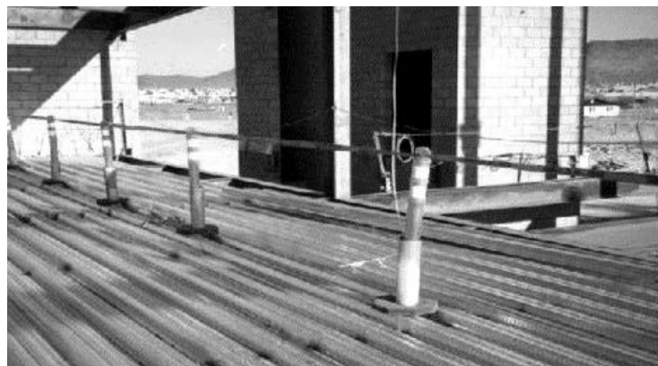
Controlled decking zone
